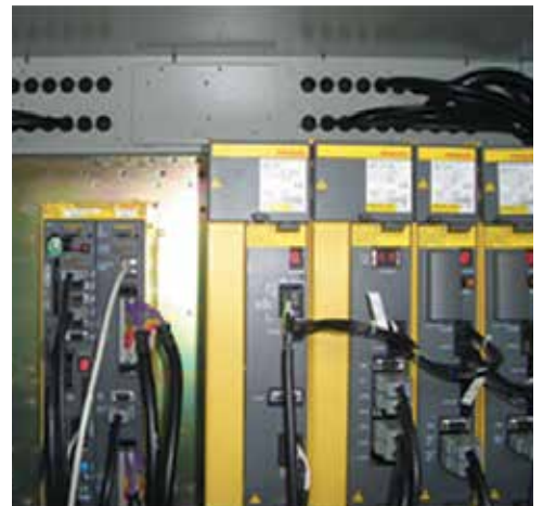
Water-proof fittings are mounted at the openings for wires to avoid invasion of oil mist.
